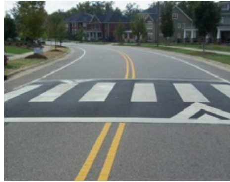
Install Raised Pedestrian Crossing
