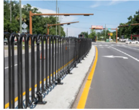
Install Pedestrian Median Fencing on Approaches
