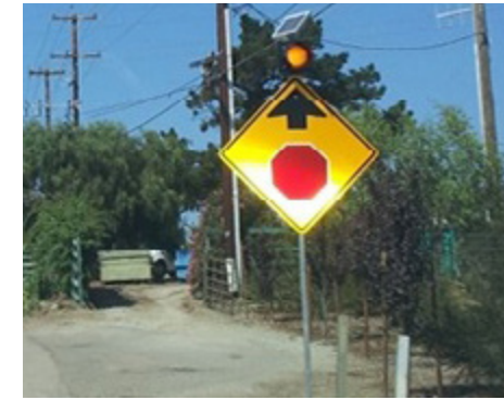
Install Flashing Beacons as Advance Warning
