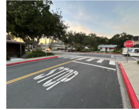
Upgrade Intersection Pavement Markings
