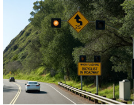
Install Curve Advance Warning Signs (Flashing Beacon)
