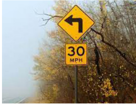
Install Curve Advance Warning Signs
